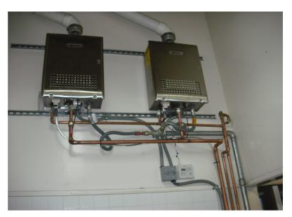
The old tank was well beyond its useful life (around 5-7 years in a commercial setting). It was also very inefficient. Woodside Priory contacted Tanknot Tankless, Inc. to assess the equipment and recommend an upgrade. Two Noritz NCC199's were installed with a capability of 600 gallons per hour of hot water. In addition, much of the piping which served the kitchen was re-piped from oversized 1-1/2" pipe down to 3/4" pipe, greatly reducing hot water delay, water waste and gas loss.
